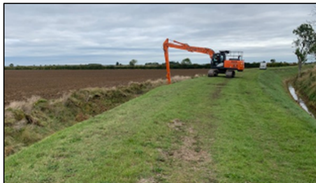
Photo 6: Work by BSIDB on the Heckington Eau
